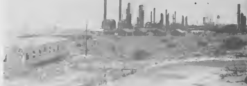
THIS UNDATED photograph shows the early Lago scene. Present day Combination and Vibreaker units occupy approximately the same area in which the pictured first processing and breakdown units were positioned. The line of stacks on the right belong to the rerun complex, of which Nos. 3, 5, 7 and 8 still are on location. The Cat Plant, which was inaugurated in December, 1943, was constructed in the area left of the existing unit. Present day Lago refinery scene, right, shows striking change.
